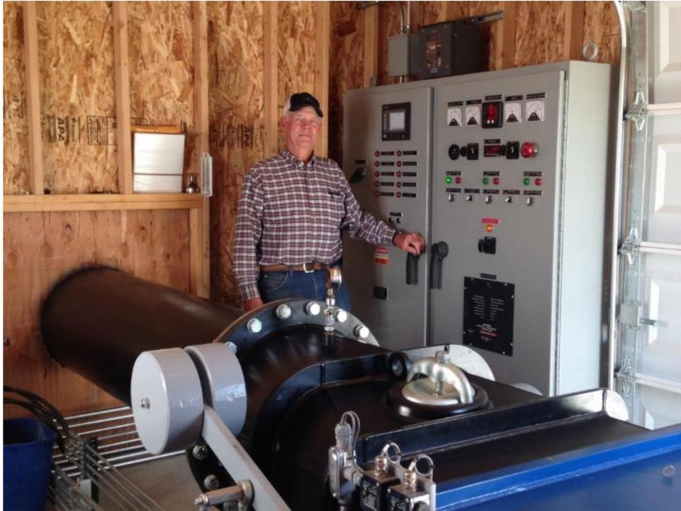
Water at Jim Park's farm is diverted into an underground penstock parallel to the ditch, where it flows into the powerhouse to spin a turbine. It returns to the ditch just below the powerhouse.
